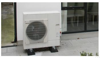
Figure 2: Air Source Heat Pump Outdoor Unit
