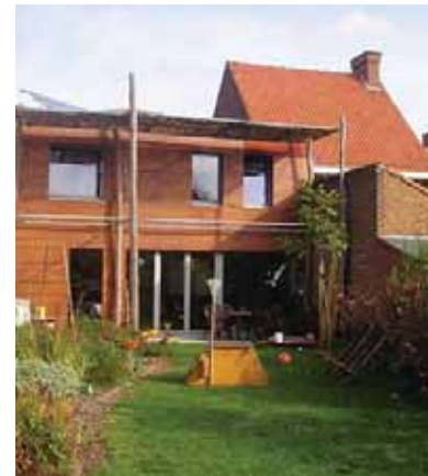
Passive house in Ghent, Belgium (2004). Source: Passiefhuis Platform vzw.
