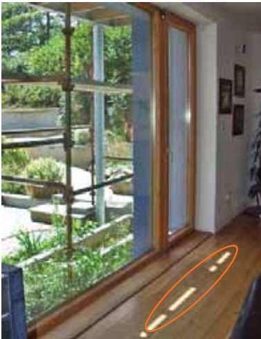
Photo depicting how the house is shaded from the high summer sun by the overhang/awning/balcony. Source: MosArt Architecture.
