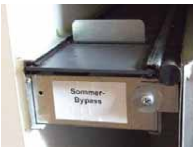
The sommer-bypass can be used for cooling in the summer if needed. Source: MosArt Architecture.
