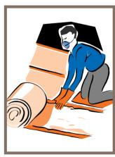
To ensure that there is adequate ventilation at the eaves, cut the ends of the insulation in a wedge shape. Alternatively buy specially shaped plastic eaves pieces to ensure that the insulation does not block the eaves ventilation.
