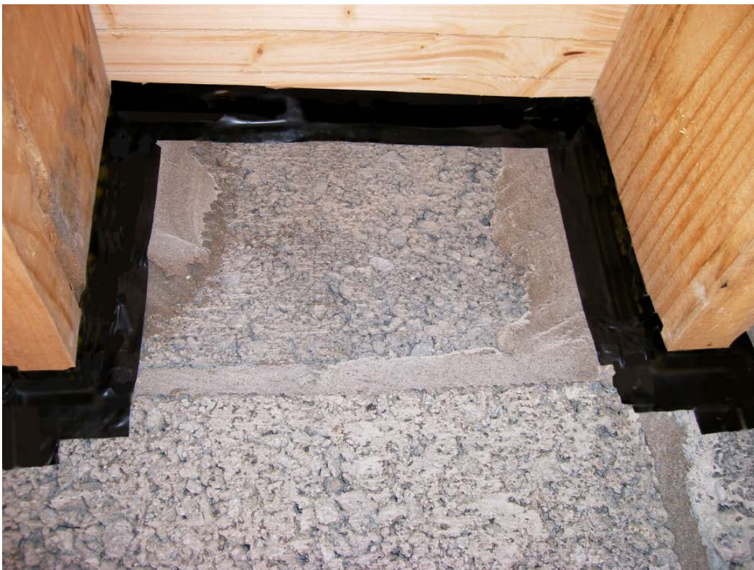
Figure 10 Sealing at intermediate floors: Second stage: tape joists to wall
