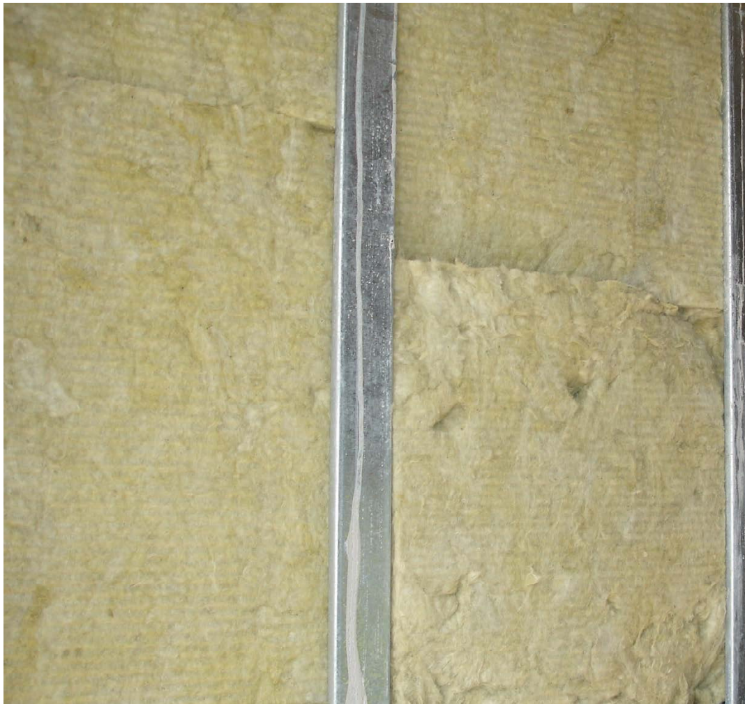
Figure 7 Tightly-fitting insulation in lightweight frame
