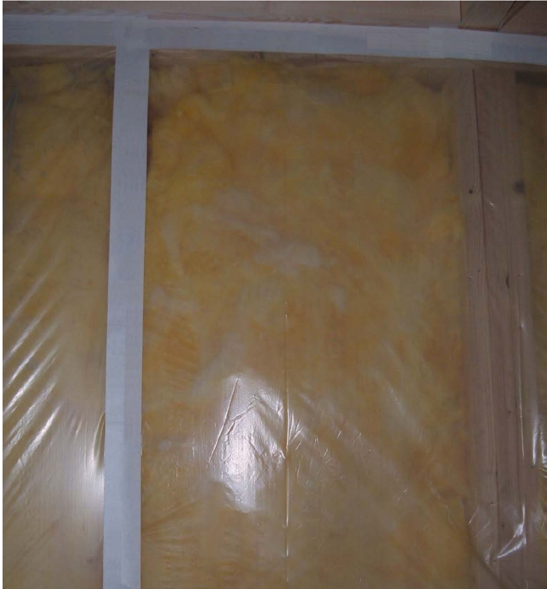
Figure 8 Joints sealed in air tight membrane
