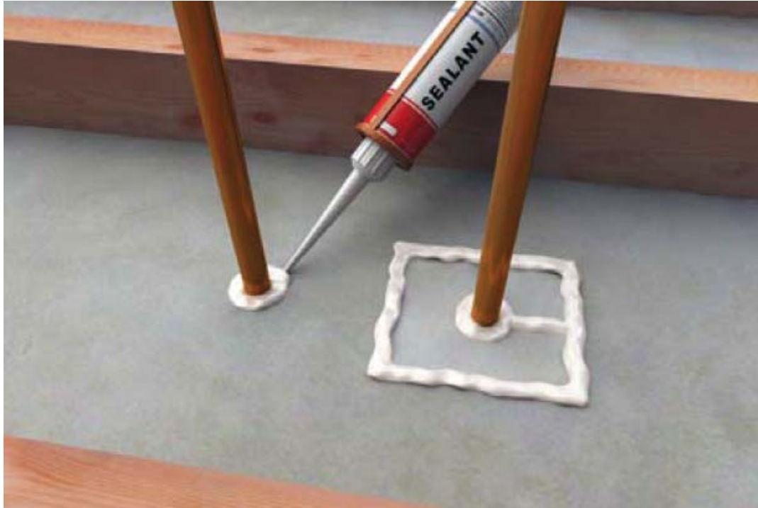
Figure 4 Sealing where pipes enter the roofspace
