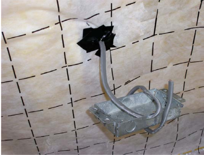
Figure 13 Sealing around connection to electrical socket outlet
