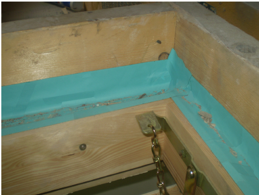
Figure 15 Sealing around frame of access hatch to attic
